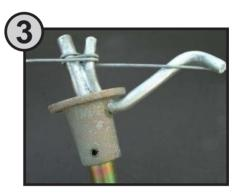
Lock Klaw Klip over wire to prevent unwinding.
